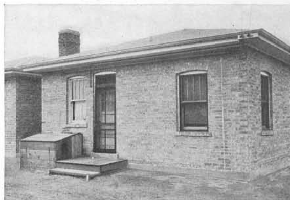
Rear Wall of a Garlow Showing 18 Ft., Built-in Steel Beam Construction. The brick beneath the beam is built into a panel which can be removed without disturbing the rest of the wall. This leaves a space for swinging the garage doors.
